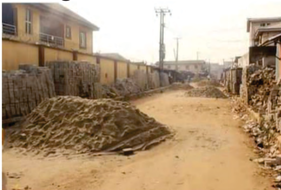
Ongoing rehabilitation of James Okiki Road
